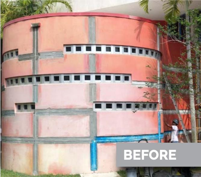
After five years in the hot Florida sun, the paint on the building's exterior had faded, chalked and deteriorated.
